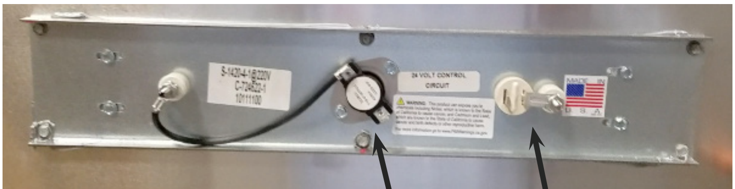
Automatic Over Temperature Control Switch (AOTC) Fusible Link
