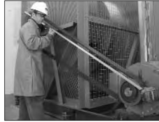
Using a straight edge to check alignment
