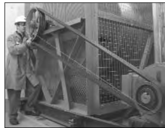
Using a string to check alignment
