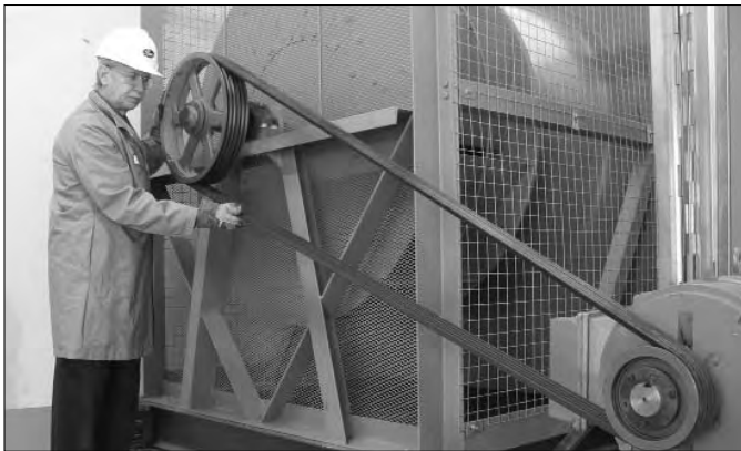
Begin by inspecting the belt
